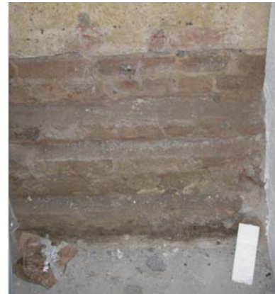
Footing to be Underpinned (Figure 8)
