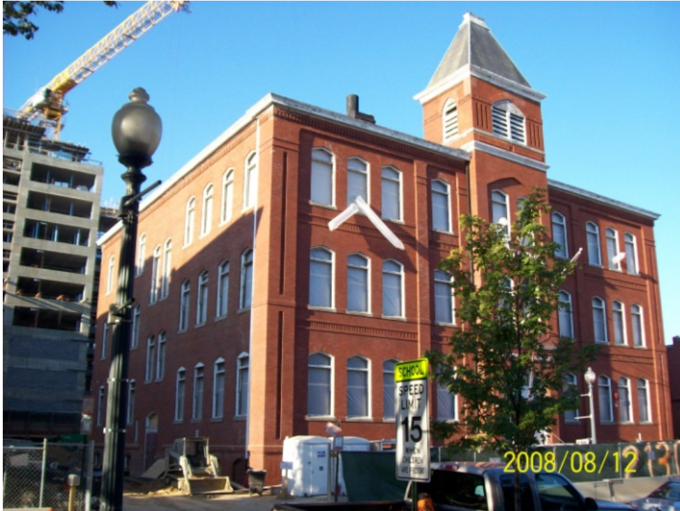
Pre-modernization and Addition (Figure 2)
